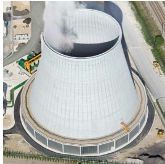
Fan Assisted Natural Cooling Tower in the Ribatejo power plant in Portugal
