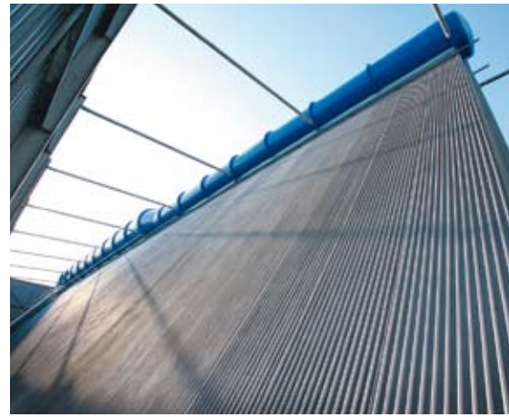
Inside view of the Alex Air Cooled Condenser
